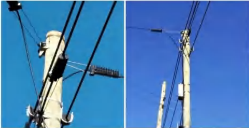
1.Suspended from a hook bolt The clamp can installed on a 14mm ~ 16mm hook bolt on wood poles. 2.Secured with pole banding The clamp be installed on wood poles, round concrete poles, and polygonal metallic poles using one or two 20mm pole bands 3.Bolted The clamp can be secured with a 14mm ~ 16mm bolt on wood poles.
